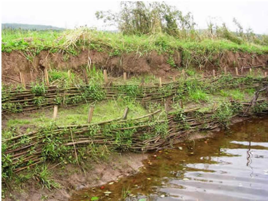
Figure 12-14. Wattle Fences ( http://www.kennebecasisriver.ca/wattle.html )
