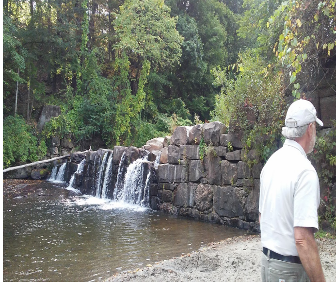
Figure 7-20: From initial site visit in Sep. 2017; shows no water flowing through right hand portion of the dam
