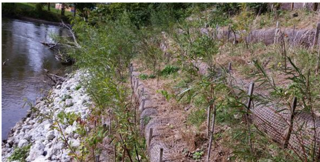
Figure 12-5. Live Staking
