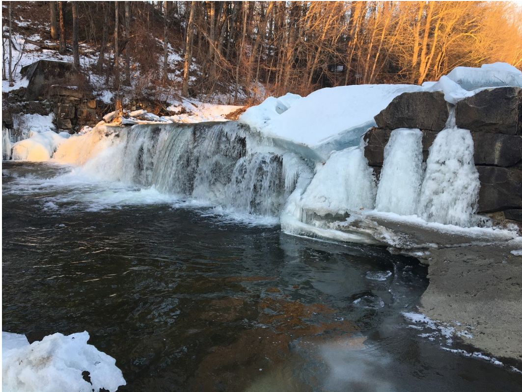
Figure 7-19: Water flowing through Dam cracks
