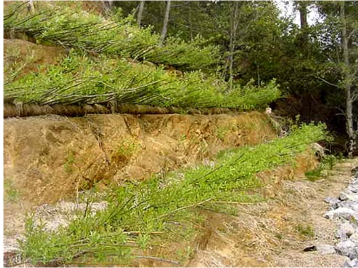
Figure 12-9. Brush Layers ( https://www.dec.ny.gov/docs/water_pdf/sec4.pdf )
