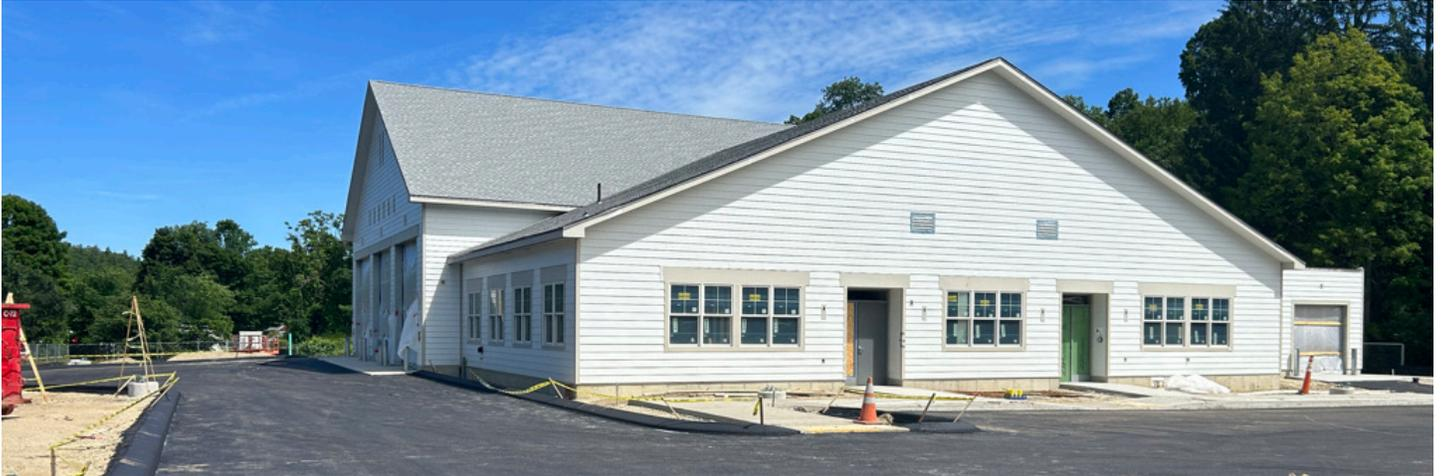
In the past couple of months, the project has reached significant milestones. Most noticeable is the parking lot and curbing. The first layer of asphalt binder is in and the majority of the concrete sidewalks and entries have been completed. The stormwater retention beds are in progress. In the next month we should see more finish site work including the removal of the site trailer and restoration of the green space at the corner of Main and South Streets.
