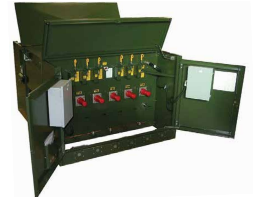
Figure 1. VFI underground distribution switchgear offers a simplified approach to the protection of 15, 25, and 35 kV underground systems, and provides a wide choice of switching combinations to meet system requirements.
