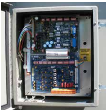
Figure 6. TPG control with SCADA shown.
