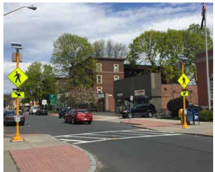
Rectangular Rapid Flash Beacon (RRFB) in West Springfield
