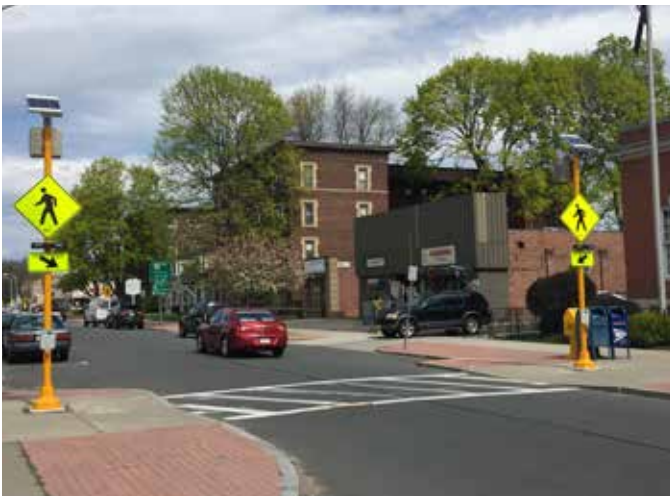
Rectangular Rapid Flash Beacon (RRFB) in West Springfield
