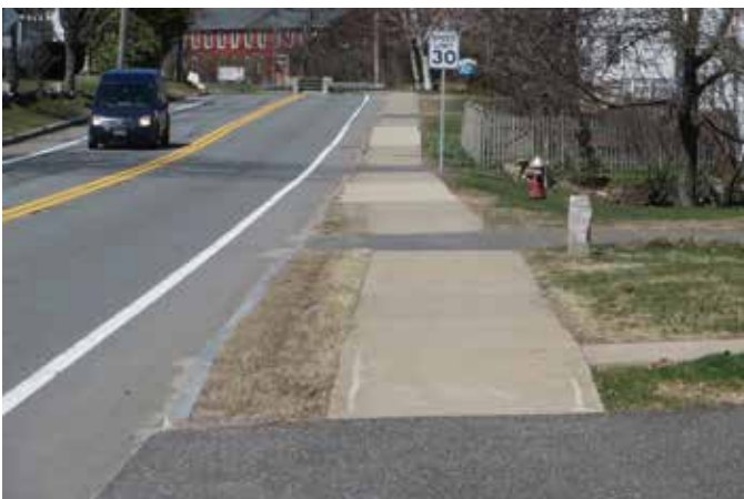
Route 9 corridor looking west toward Buttonshop Road
