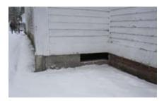
The fieldstone foundation has openings to the outdoors. It may be susceptible to movement by frost. Dirt floor in the crawlspace is allowing moisture to attack the floor structure.
