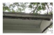
Soffits have significant rot. Gutters have also failed.
