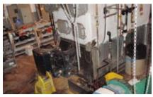
The boiler is well beyond its service life and could break down at any time.
