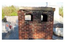
The chimney is badly cracked and in need of rebuilding.
