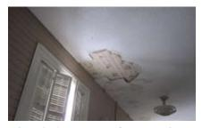
Though the main roof is in good condition, water is getting in around the cupola, resulting in damage to the building and the collection of the Historical Society housed inside.
