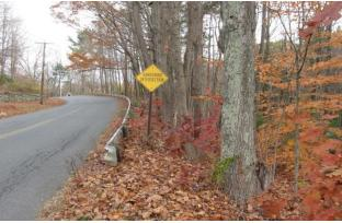
**Concern:** No advanced warning signage for side road intersection located on a curve.
