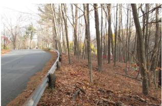
**Concern:** Deteriorated guard rail posts and poor guard rail condition.
