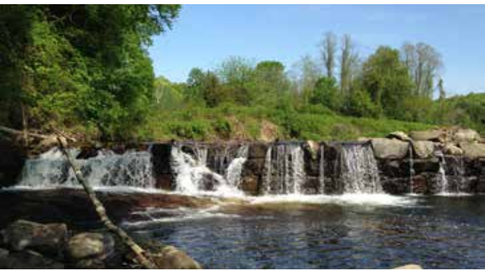
Damaged by storms, the dam is perhaps half its original height, and what remains of the former pond is filled with sediment. Much of the original pond area is growing in with vegetation.
