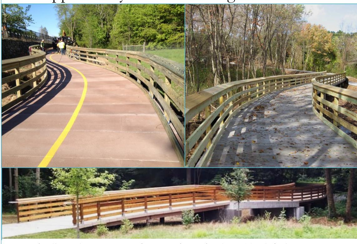
Boardwalks with concrete surfacing and wood railings. Top left shows concrete boardwalk with shallow footings in Hadley, MA on the Norwottuck Rail Trail. Boardwalk images from PermaTrak.
