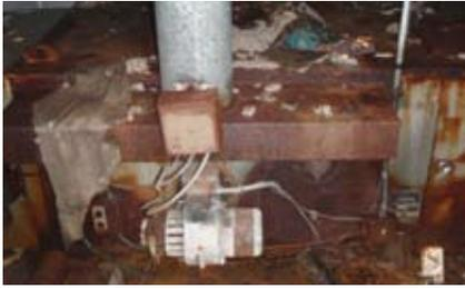
*The building is not heated. Its boiler has not been functional for years.*
