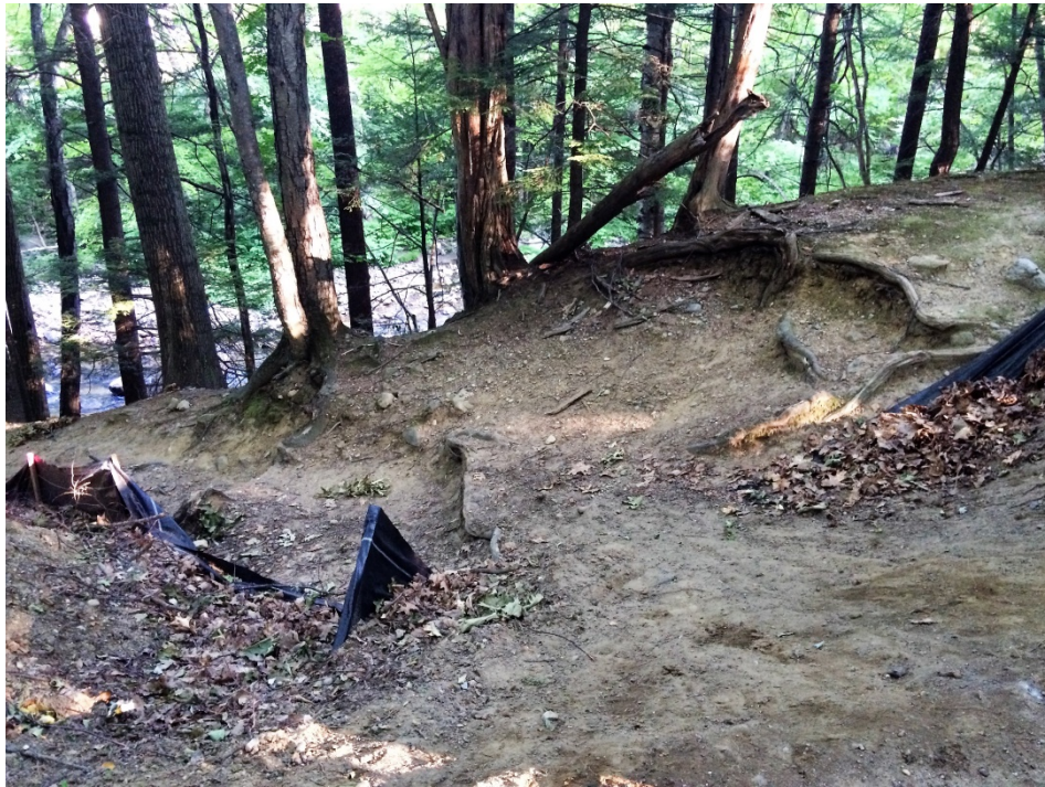
Photo 1: Photo looking north taken from rail trail looking at entrance to “goat path” dismount, Mill River in background on left side of photo. Trail has been eroded and incised.
