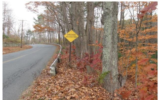
**Concern:** No advanced warning signage for side road intersection located on a curve.
