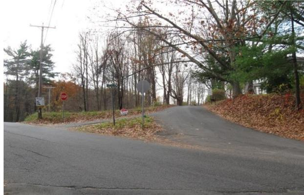
**Concern:** Poor intersection alignment with poor sight distance.
