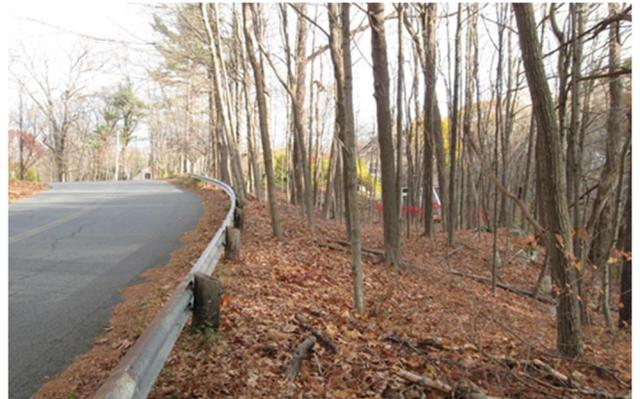
**Concern:** Deteriorated guard rail posts and poor guard rail condition.
